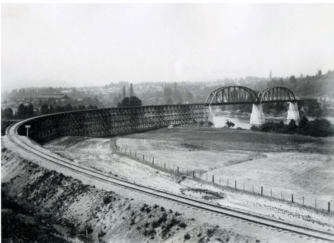
The approach appears on the left side of the bridge in this photo
